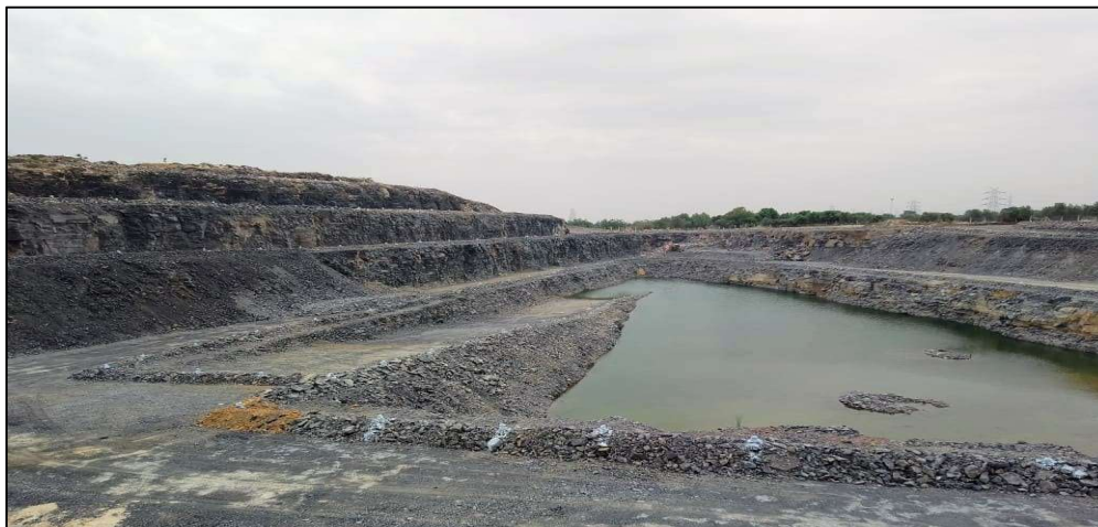
Rain Water Harvesting Pit at Mines area
