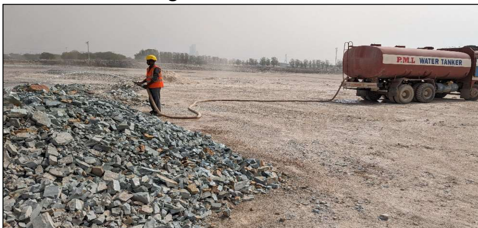
Muck Pile Wetting
