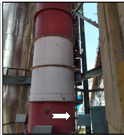
Coal Mill Stack
